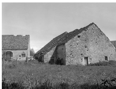
Pignon droit. Phot. Yves Sancey IVR43_19813900045X
