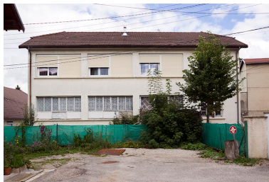
Façade antérieure. Phot. Yves Sancey IVR43_20132501788NUC2A
