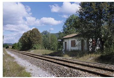
Abri - lampisterie. Phot. Yves Sancey IVR43_20043900362ZA
