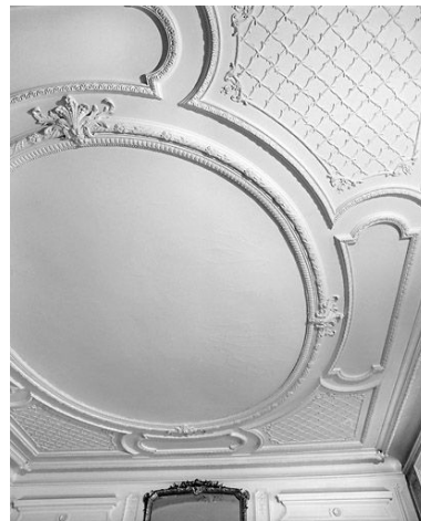
Grand salon : plafond. Phot. Yves Sancey IVR43_20033900817X
