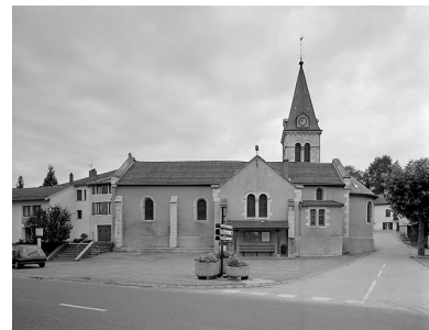
Face sud. Phot. Yves Sancey IVR43_19963900848V
