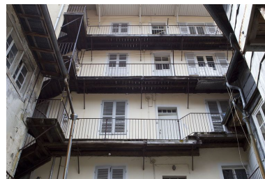
Coursières. Phot. Yves Sancey IVR43_20103900167NUC2A
