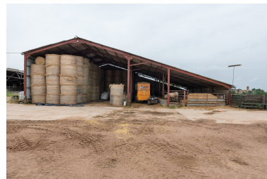
Hangar agricole. Phot. Pierre-Marie Barbe-Richaud IVR26_20187100214NUC4A
