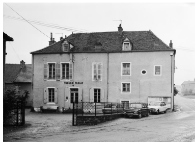
Façade principale. Phot. Jean-Luc Duthu IVR26_19802100249V
