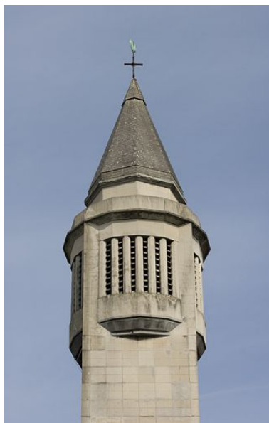
Clocher. Phot. Yves Sancey IVR43_20062500711NUCA
