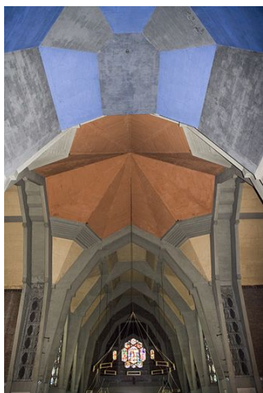
Plafond du transept. Phot. Yves Sancey IVR43_20062500691NUCA
