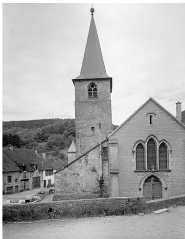
Façade antérieure. Phot. Yves Sancey IVR43_19853900230V
