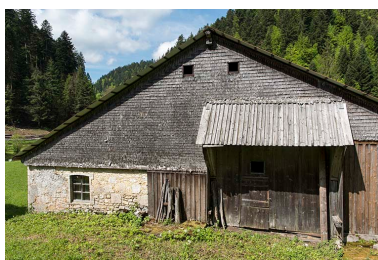
Façade postérieure. Phot. Sonia Dourlot IVR43_20172500679NUC4A
