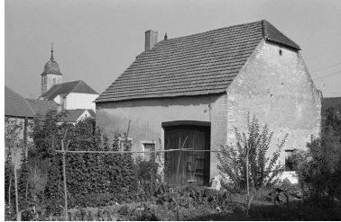
Logement patronal (A). Phot. Laurent Poupard IVR43_19883900565Z
