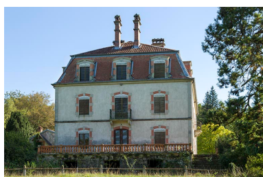
Façade nord. Phot. Sonia Dourlot IVR43_20157000685NUC2A
