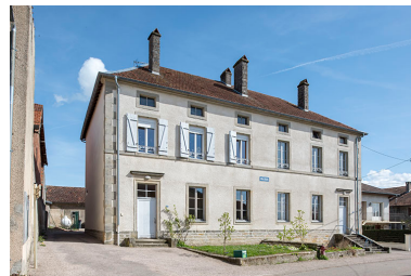
La mairie. Phot. Sonia Dourlot IVR43_20177000326NUC4A
