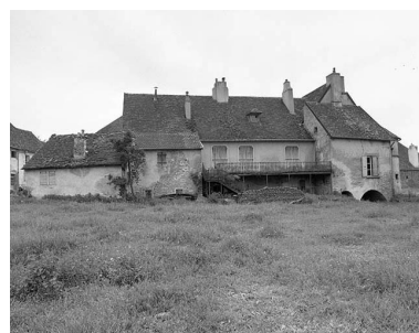
Façade nord. Phot. Yves Sancey IVR43_19813900182X
