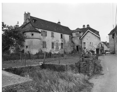
Façade ouest. Phot. Yves Sancey IVR43_19813900177X
