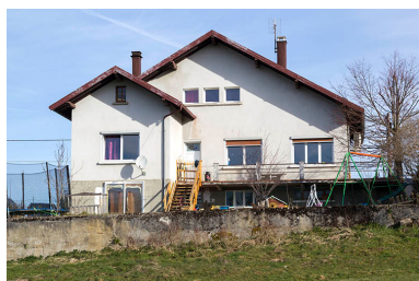
Façade postérieure. Phot. Sonia Dourlot IVR43_20152500778NUC2A
