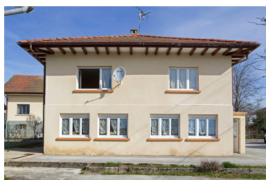
Façade postérieure. Phot. Sonia Dourlot IVR43_20152500866NUC2A
