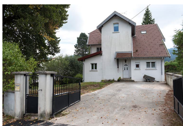
Façade antérieure. Phot. Sonia Dourlot IVR43_20162501355NUC4A
