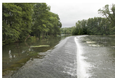
Le barrage. Phot. Jérôme Mongreville IVR43_20097000671NUC2A
