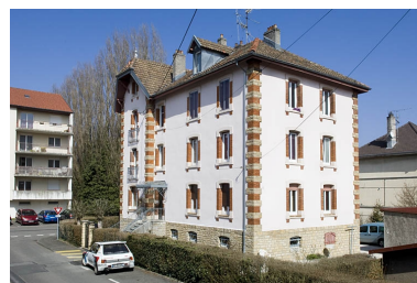
Habitation collective (?). Phot. Marc Loukachine IVR43_20122500265NUC2A
