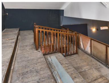
Balcon. Phot. Pierre-Marie Barbe-Richaud IVR26_20255800025NUC4A
