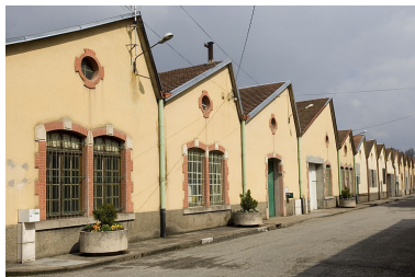
Pignons de sheds. Phot. Jérôme Mongreville IVR43_20067000146NUCA
