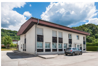
Administration, façade postérieure. Phot. Jérôme Mongreville IVR43_20143900477NUC4A
