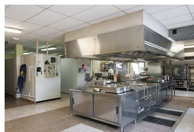
Restauration : cuisines Phot. Jérôme Mongreville IVR43_20143900506NUC4A
