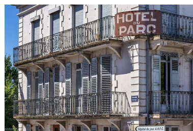
Façade est, balcons. Phot. Jérôme Mongreville IVR43_20207000574NUC4A
