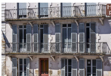
Façade est, balcons. Phot. Jérôme Mongreville IVR43_20207000575NUC4A
