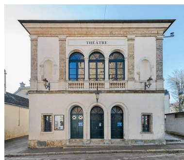
Façade antérieure. Phot. Pierre-Marie Barbe-Richaud IVR26_20222100362NUC2AQ
