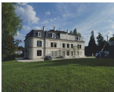
Façade nord. Phot. Yves Sancey IVR43_20029000260XA
