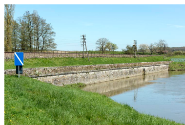
Digue ferroviaire. Phot. Sonia Dourlot IVR43_20167000313NUC4A
