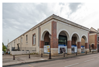
Centre Vulabelle. Phot. Pierre-Marie Barbe-Richaud IVR26_20248900066NUC4A
