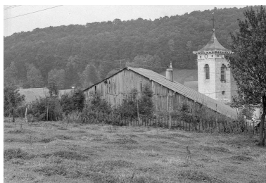
Façade postérieure. Phot. Gilbert Poinot IVR43_19752501366Z
