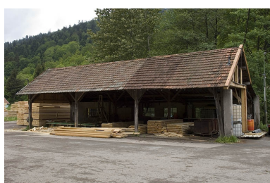
Magasin industriel. Phot. Jérôme Mongreville IVR43_20067000412NUCA
