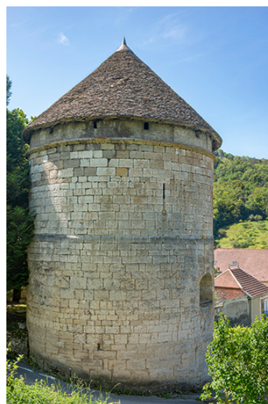
Elévation nord. Phot. Jérôme Mongreville IVR43_20243900849NUC4A
