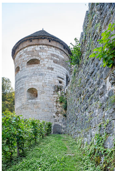
Elévation ouest. Phot. Jérôme Mongreville IVR43_20243900861NUC4A
