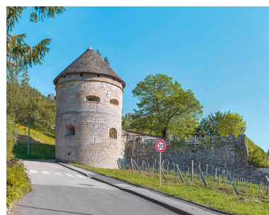
Elévation nord. Phot. Thierry Kuntz IVR43_20223900614NUC4A
