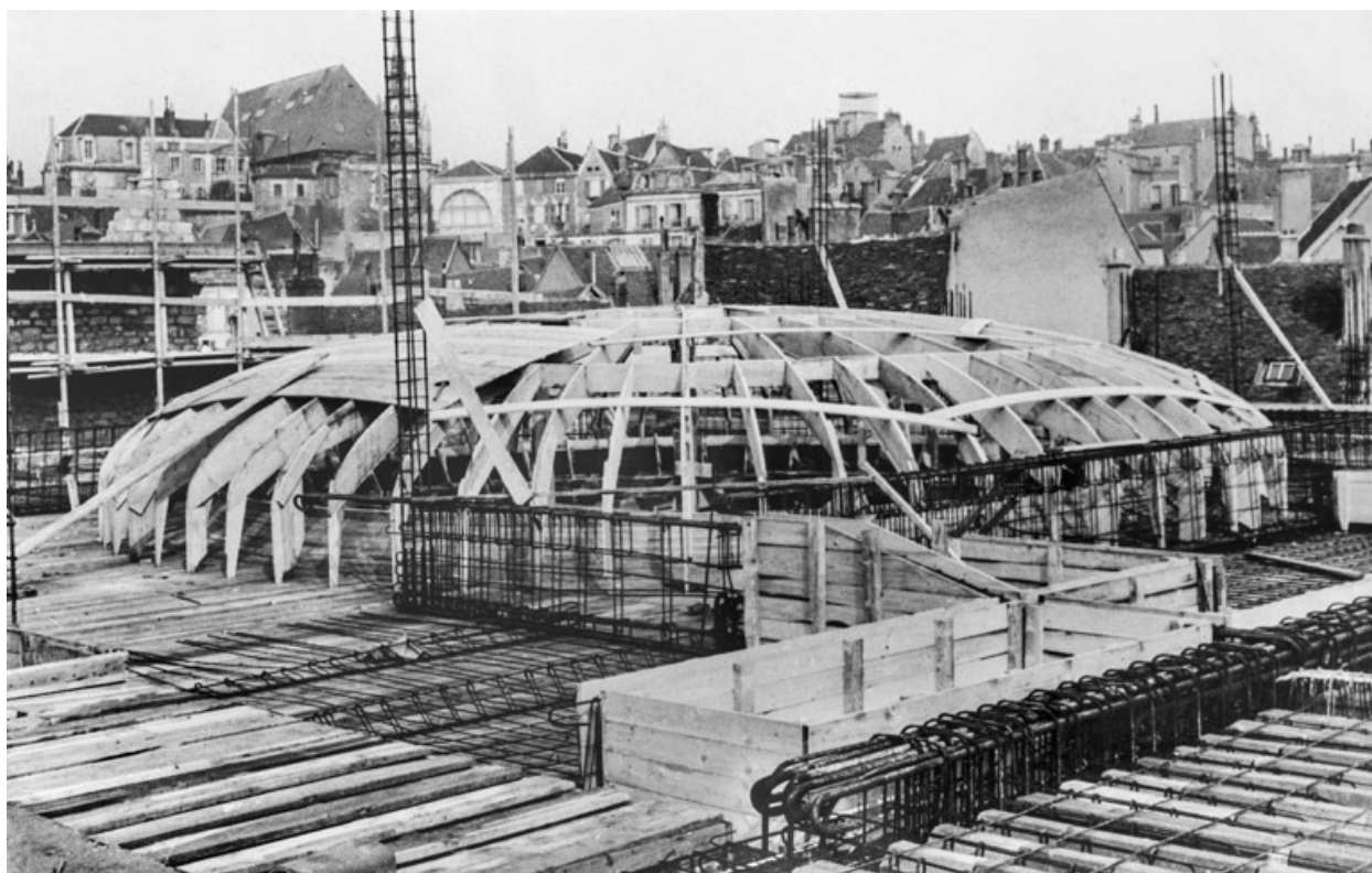
[La coupole en construction]. S.d. [1938].
