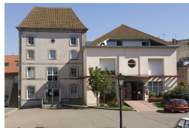
Bureaux (?). Phot. Jérôme Mongreville IVR43_20067000847NUCA
