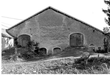
Façade postérieure. Phot. Yves Sancey IVR43_19802500907X
