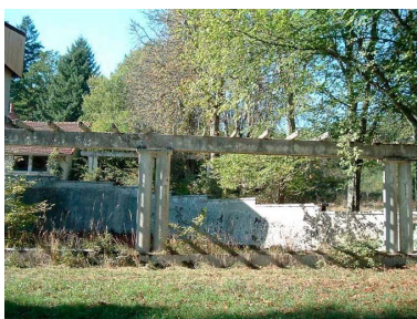
Pergola. Phot. Sylvie Le Clech-Charton IVR26_20052101996NUCA
