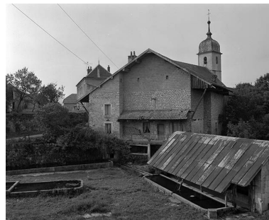
Elévation du logis. Phot. Yves Sancey IVR43_19802500881X
