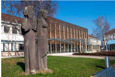
Vue de profil. Phot. Mary Ruffinoni IVR43_20142500036NUC4A
