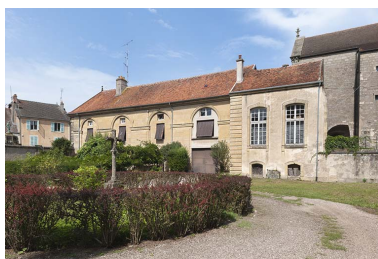
La cour. Phot. Mary Ruffinoni IVR43_20127000345NUC4A
