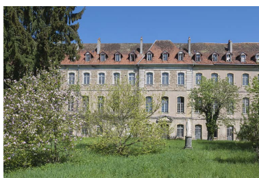
Façade sud vue de face. Phot. Mary Ruffinoni IVR43_20137000021NUC4A
