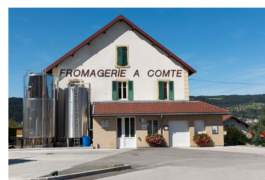
Façade antérieure. Phot. Sonia Dourlot IVR43_20172501813NUC4A
