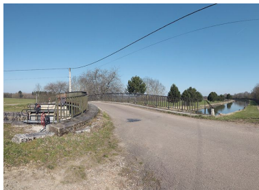
Le pont. Phot. Thierry Kuntz IVR26_20122102737NUC4A
