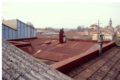
Toiture. Phot. Yves Sancey IVR43_19943900834ZA
