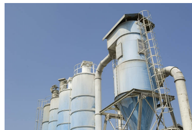
Silos. Phot. Jérôme Mongreville IVR43_20097000765NUC2A
