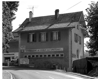
Façade nord. Phot. Yves Sancey IVR43_19973901229X
