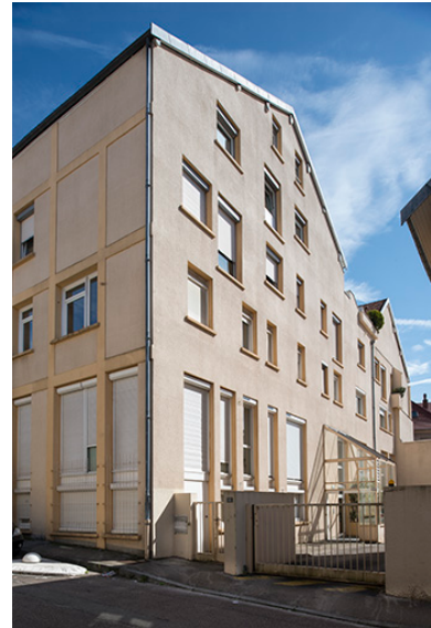
Mur-pignon ouest. Phot. Jérôme Mongreville IVR43_20172501173NUC4A
