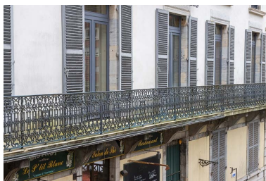
Façade nord, balcon. Phot. Jérôme Mongreville IVR43_20223900313NUC4A
