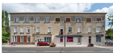
Vue de face. Phot. Pierre-Marie Barbe-Richaud IVR26_20205800479NUC4AQ
