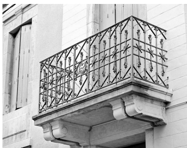
Balcon. Phot. Yves Sancey IVR43_20033900216X
