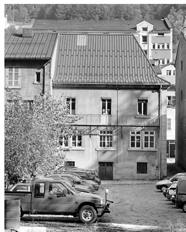
Façade postérieure. Phot. Yves Sancey IVR43_20033900214X
