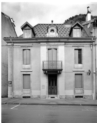
Façade antérieure. Phot. Yves Sancey IVR43_20033900213V
