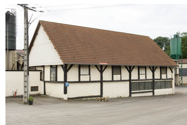
Magasin industriel. Phot. Jérôme Mongreville IVR43_20087000712NUC2A
