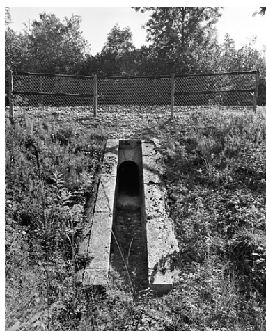
Aqueduc. Phot. Yves Sancey IVR43_20050100023X
