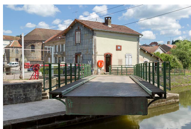
Pont en rotation. Phot. Sonia Dourlot IVR43_20157000989NUC2A
