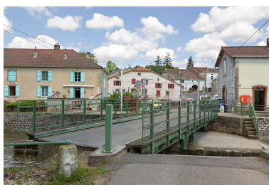
Pont en rotation. Phot. Sonia Dourlot IVR43_20157000990NUC2A
