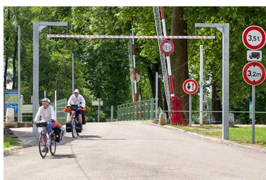
Cyclistes franchissant le pont. Phot. Sonia Dourlot IVR43_20157000999NUC2A
